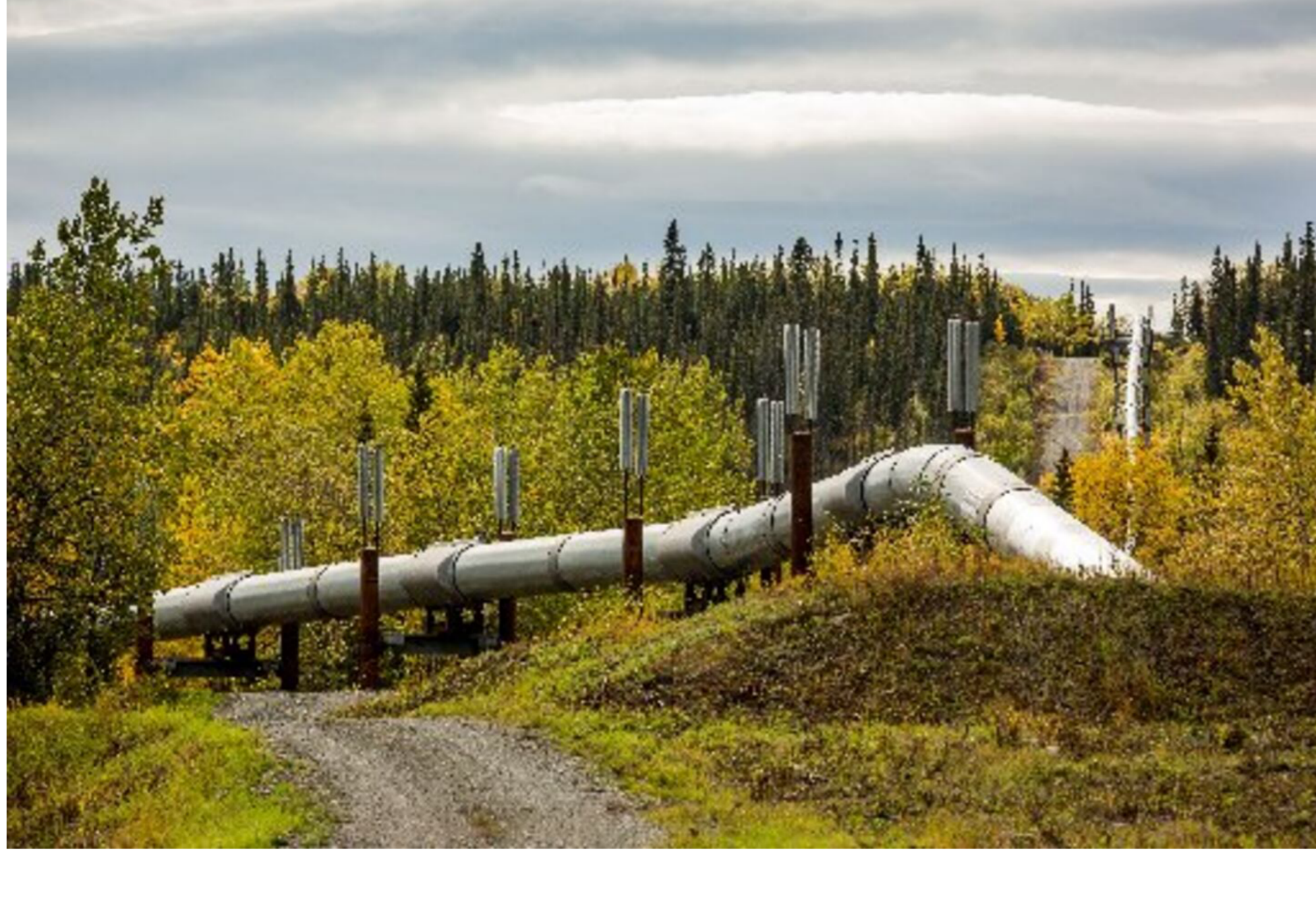
The trans-Alaska Oil Pipeline near Copper Center in September 2014. (LOREN HOLMES/ADN archive 2014)
